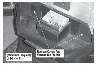
Figure 43 - Accessing Ash Clean-Out Ports – Profile 30 Series
